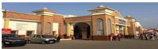
Figure 2.1.4 Bareilly Jn. Railway Station (Source:Author)
