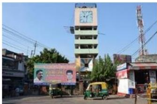
Figure 2.2.6 Clock tower, Bareilly
